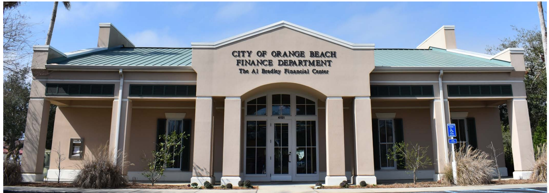
Finance Department Office on Hwy 161
